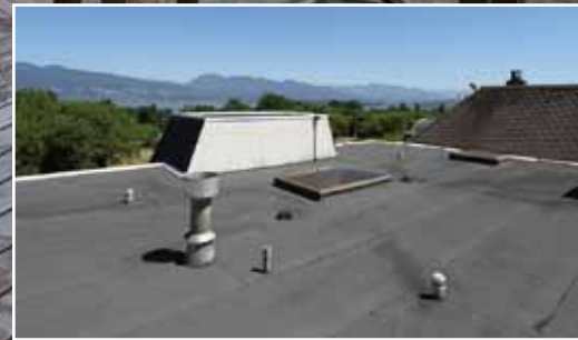
As part of a whole house renovation, My House Design Build of Surrey, B.C. converted a boring house roof into hundreds of square feet of flat rooftop seasonal living space.
