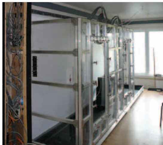
Figure 2: Interior of finished ICF walls and the climate control enclosure.
