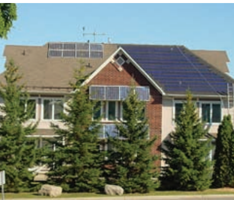
A roof-integrated PV system is being installed at the InfoCentre of the Canadian Centre for Housing Technology, and will be evaluated for durability, air leakage, wind loads, and water penetration.
